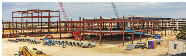
Construction continues at the Apple campus in Austin. Photo by Elizabeth
