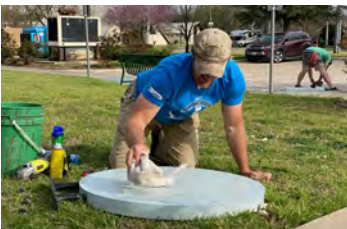
Volunteers Steph Lewis, Lisa Bailey, and Lee Harle stripping the old, cracked adhesive off the Downtown Parking signs in preparation to be resurfaced.
